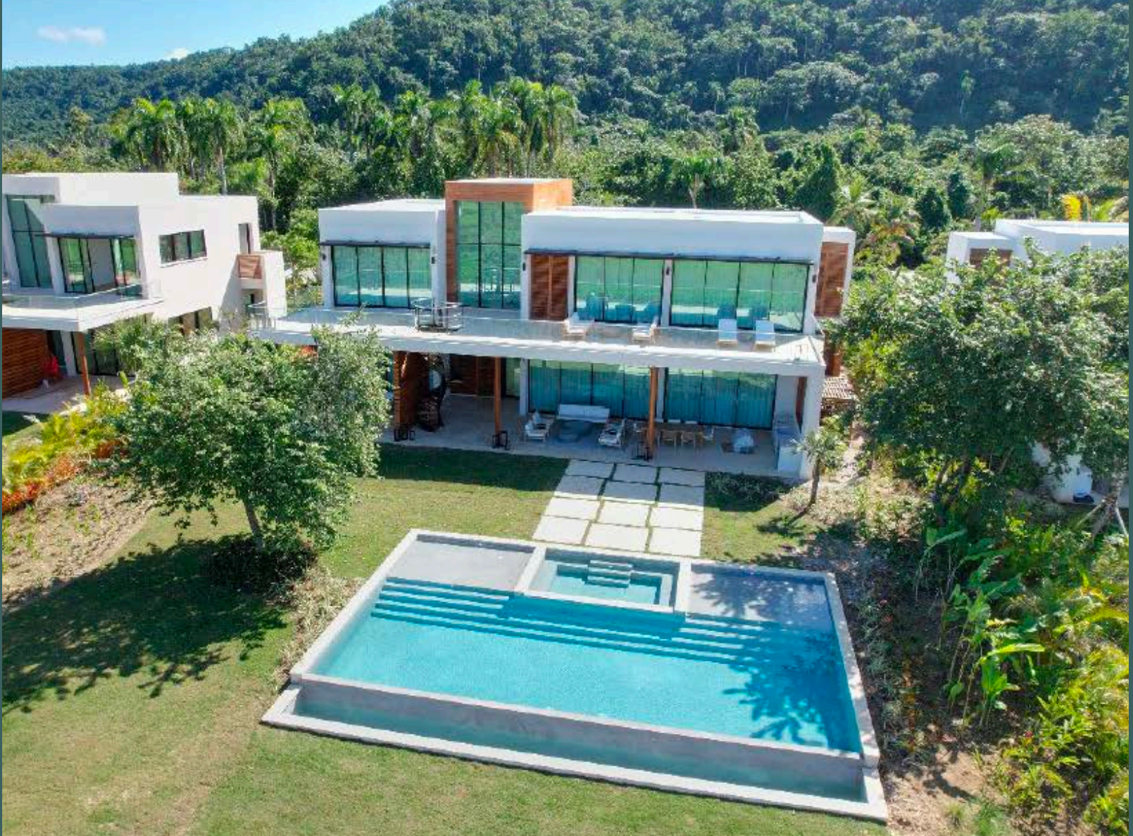
Rear Aerial View
